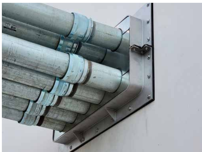
Stainless steel flange split for subsequent dowelling
